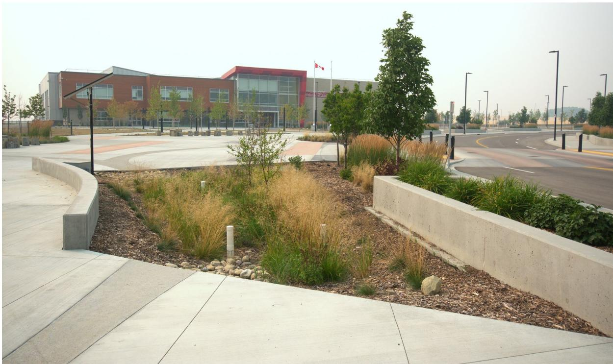
The Okotoks bioretention/storage chamber 'drought resilient LID' research and demonstration project directs runoff from a parking lot through a bioretention area and stores runoff in arch-style underground chambers, for later luxuriant landscape irrigation of a school open space. Funded in part by AEPA's WRRP. (Photo courtesy Magna Engineering)
