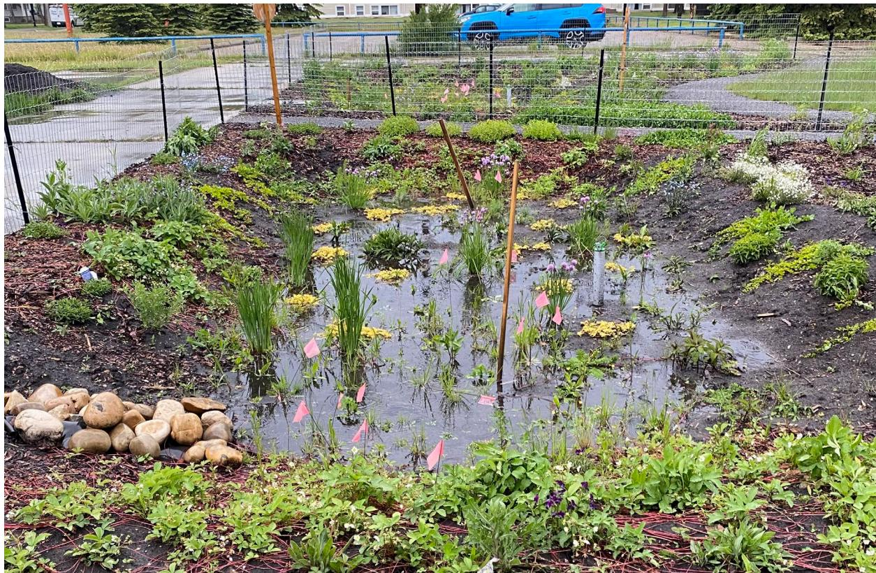
The North Glenora Resilient Landscaping Demonstration and Research project in Edmonton is a paired study of a rain garden with and without an underground wicking, milk-crate-type storage chamber. The photo shows newly planted gardens after an intense storm, with water fully absorbed in 20 minutes. Runoff is collected from the community rink shack. Funded in part by AEPA's WRRP.
