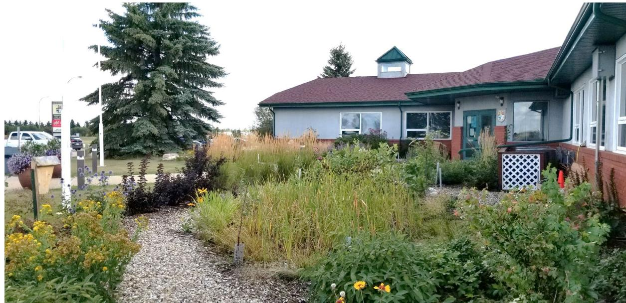
The County of Wetaskiwin administrative offices entrance was converted from a windswept heat trap that also caused nuisance flooding in the adjacent parking lot into a mini-wetland (foreground) and rain garden (background). The area quickly became an amenity space. Funded in part by AEPA's WRRP. (Photo courtesy County of Wetaskiwin)
