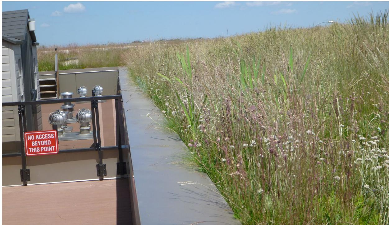
The Remington green roof in Quarry Park, Calgary is made up entirely of drought-tolerant native plants and is irrigated from parking lot runoff collected in an onsite mini-wetland that dissipates runoff through enhanced evapotranspiration on the roof. The green roof incorporates an amenity space used for social gatherings. Developer/ builder funded.
